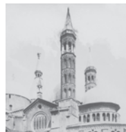
8. Padova Steeple, Basilica of Sant' Antonio
